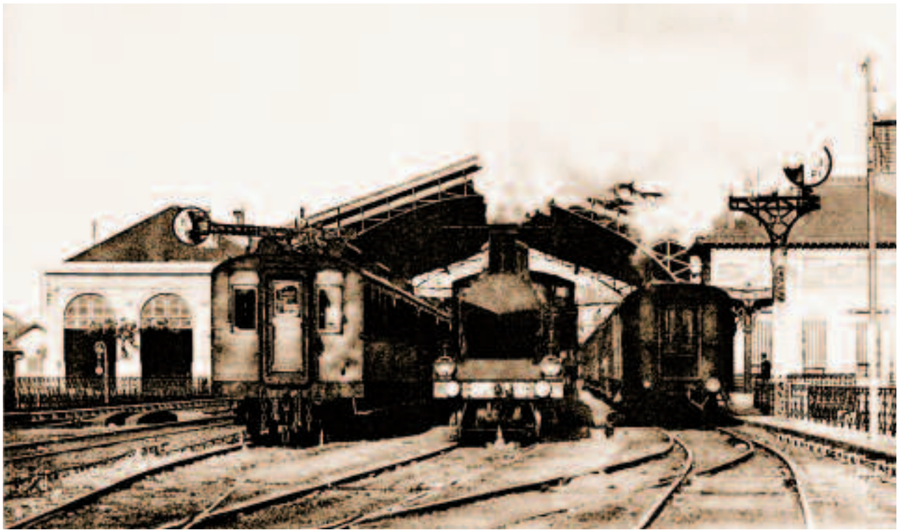
Cornavin main railway station in Geneva. Platforms for trains leaving for France.
